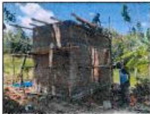
Completing the security hut for the well & pump
